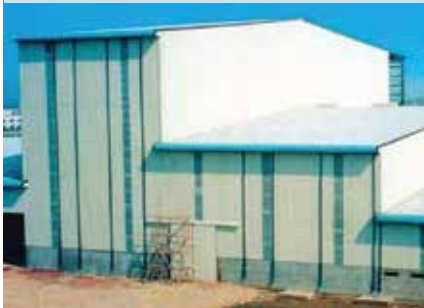
Curved Eave with Projection (without valley gutter)
