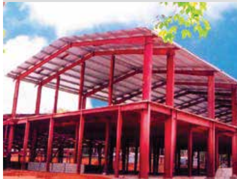
Mezzanine Floor View
