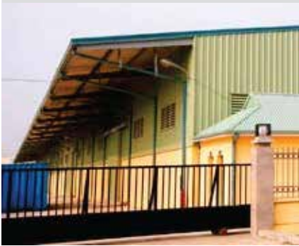
Sidewall Roof Extension
