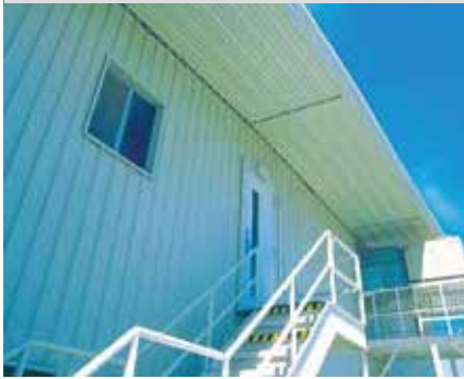
Endwall Roof Extension
